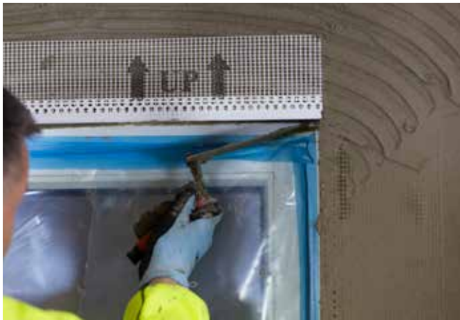
Over vindu monteres Mapetherm Dripnose Bead .
